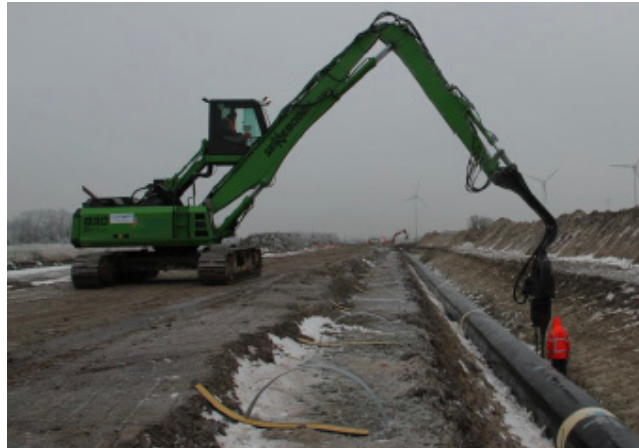
ANCHOR INSTALLATION
