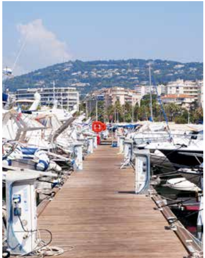
All-Concrete floats feature hardwood decking and a special mooring cleat fixing system that allows for universal adjustment.
