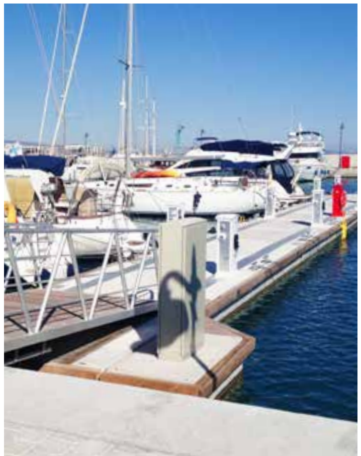
The pontoons are custom-designed Premier units with integrated open top channels and are moored by Seaflex.
