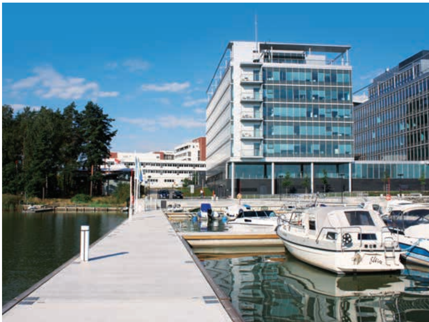
New Port Kalanokka in Finland consists of 3,3 m wide Heavy Duty pontoons, 2,4 m wide All-Concrete pontoons, Mooring Fingers and Boat Booms.
