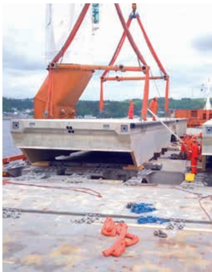
6300BRKH-series units weight 86 tons apiece with 2 x 116 ton flexible connection capacity.
