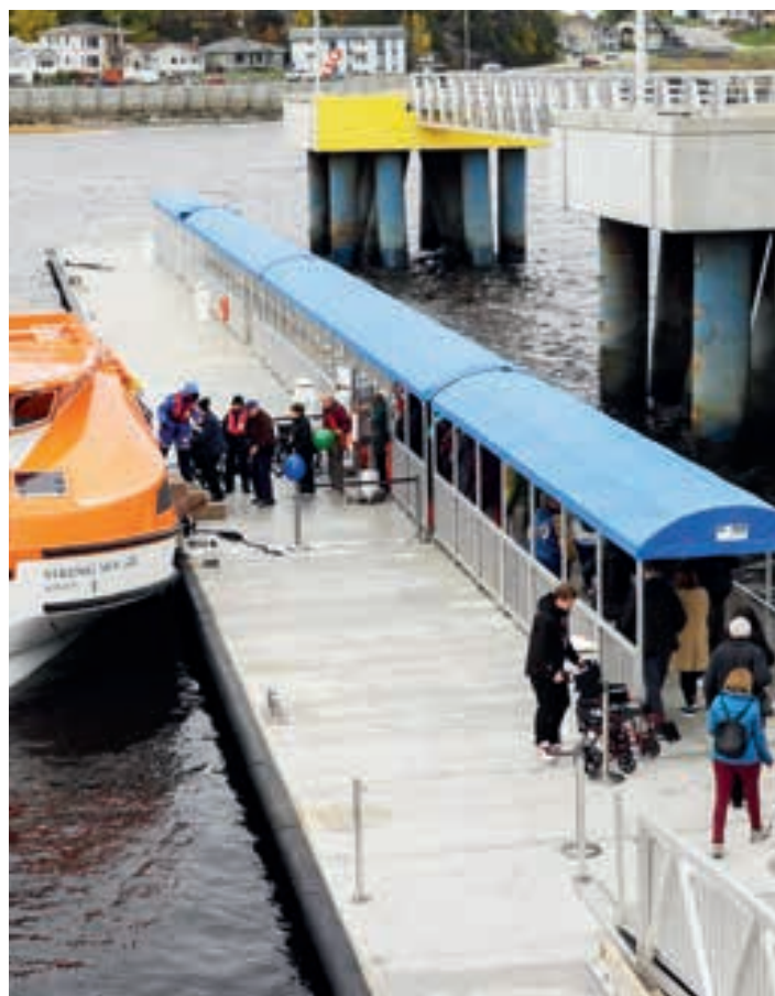
6m wide pontoons provide cruise ship passengers safe access to their shuttle vessels.
