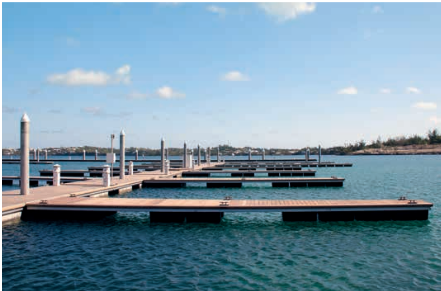
Caroline Bay Marina in Bermuda has Marinetek aluminium walkway pontoons with concrete floats and aluminium mooring finger piers with polyethylene floats.
