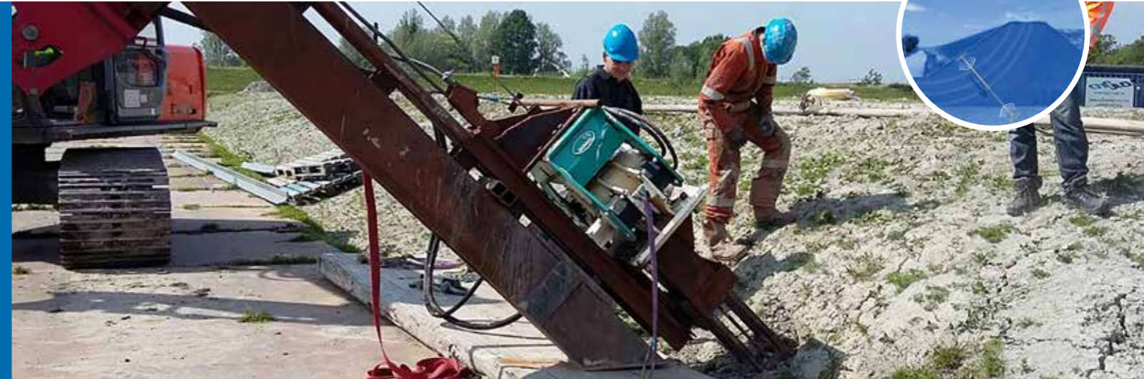
Reinforcing a test dyke.
