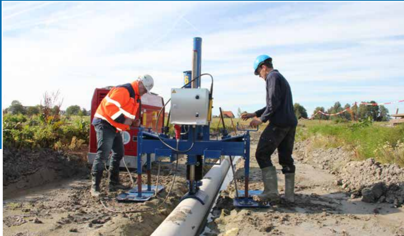
The pipeline is pushed into the soft soil in a controlled manner using light equipment.
