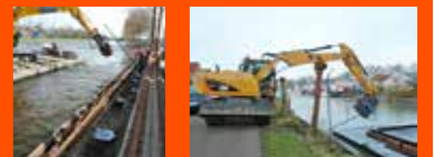
SHEET PILE ANCHORING
